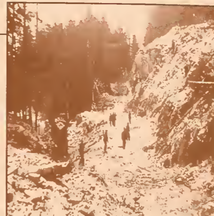
"A crew working to build road to top of mountain where station was built." Richard Pettinger
